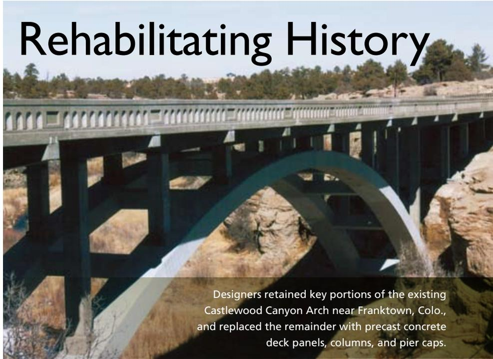
Designers retained key portions of the existing Castlewood Canyon Arch near Franktown, Colo., and replaced the remainder with precast concrete deck panels, columns, and pier caps.
