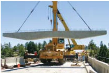
Precast concrete components of various sizes were installed due to their ease of use and rapid construction.
