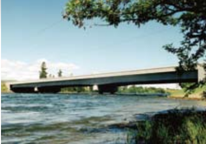
The Harvard Road Bridge near Spokane, Washington, features three precast concrete spans to minimize the number of piers. The bridge also spans the adjacent Centennial Trail.
