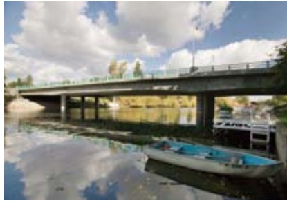
To open up the waterway, the Argonne Road Bridge features cast-in-place concrete box girders, which are used in the end spans and extend over the piers to support the precast concrete drop-in girders in the center span.
