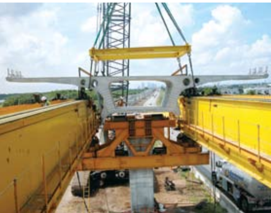
Precast concrete segments, 59-ft-wide and weighing 70 tons, were cast in a nearby facility, then delivered to the site for erection. Erection activities were timed to allow rush hour traffic on the at-grade lanes to move freely.
