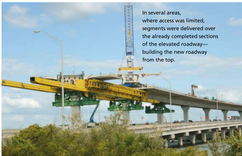
Precast concrete segments, 59-ft-wide and weighing 70 tons, were cast in a nearby facility, then delivered to the site for erection. Erection activities were timed to allow rush hour traffic on the at-grade lanes to move freely.
