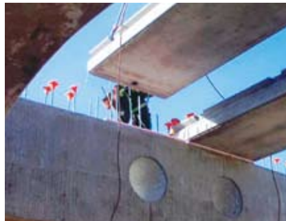
Precast concrete panels were used to replace the existing sub-deck.
