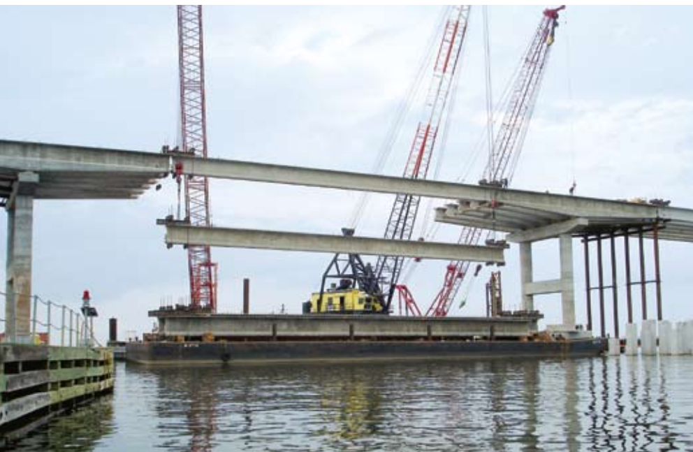
Spliced beams continue to be economical for main-span construction. Photo: PB.
