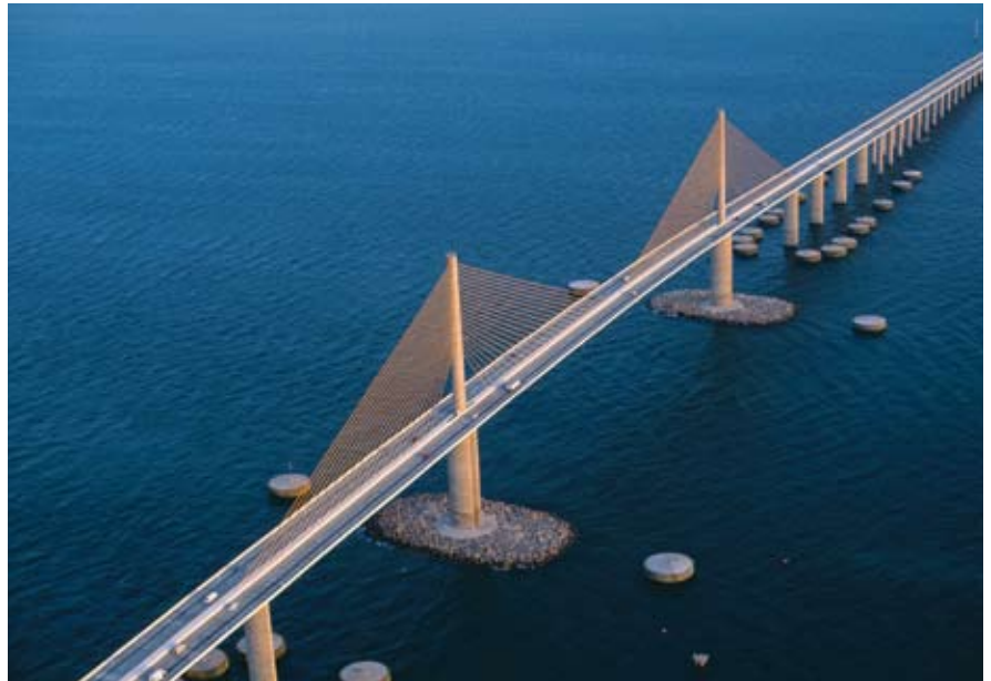
The versatility of precast segmental concrete was proven with the Skyway Bridge replacement. Photo: FIGG.
