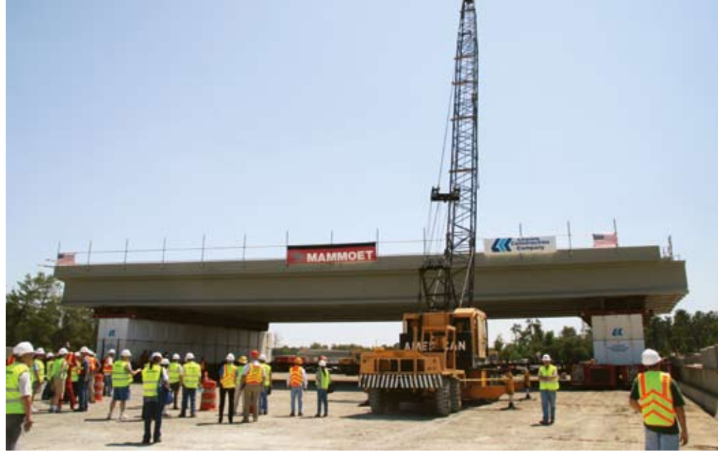
Self-Propelled Modular Transporters moved spans on land for the Graves Avenue replacement.
