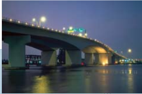
The graceful 630-ft-long span of the Acosta Bridge, in Jacksonville. Photo: T.Y. Lin International.
