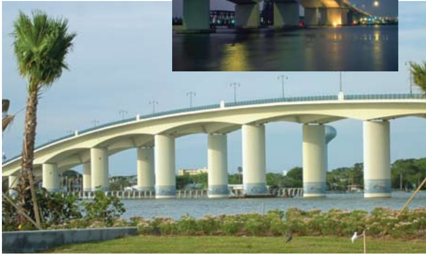
The Broadway Bridge pleases both an engineer's and an artist's eye. Photo: FIGG.
