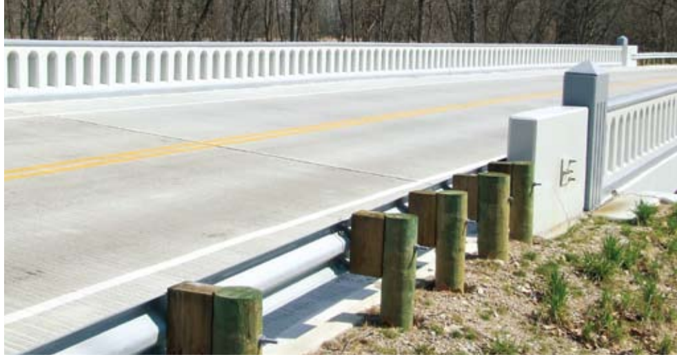
The new bridge provides ample space for vehicles, pedestrians, and bicycles.
