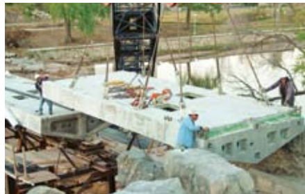
Match-cast segments are being used for the cable-stayed pedestrian bridge.
