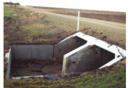
Precast concrete box culverts provide fast construction, economy, and erosion prevention.
