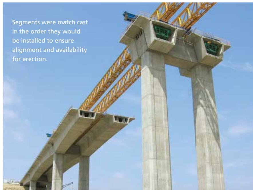
Segments were match cast in the order they would be installed to ensure alignment and availability for erection.
