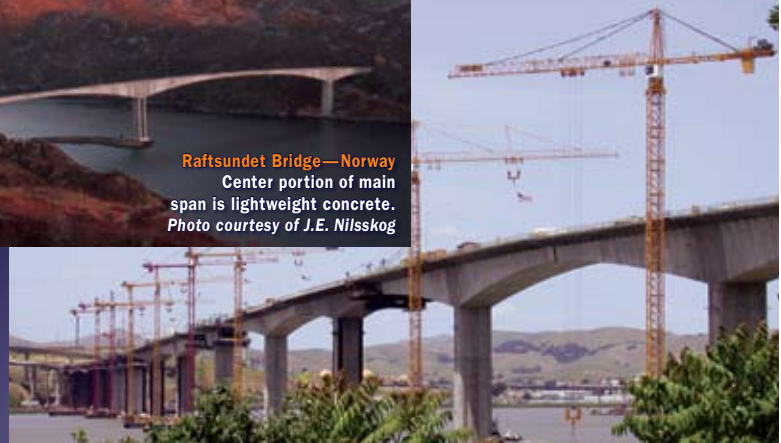
Benicia-Martinez Bridge—California Lightweight concrete box girder superstructure.
