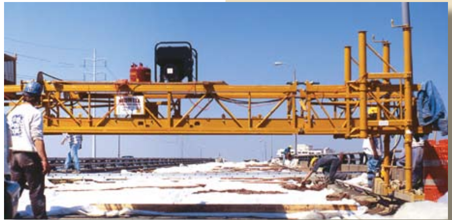
At least 7 days of curing with wet burlap and plastic sheeting are essential for bridge decks.
