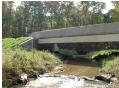
*Most of the county's bridges, like the MB Road Bridge, use adjacent box beams with composite concrete deck.*
