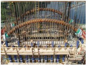
Two of the cradles positioned within the pylon are shown prior to casting. The 20 cradles in each of the pylons carry the strands (from 41 to 73 per stay) through the pylon, eliminating the need for anchorages within the pylon.
