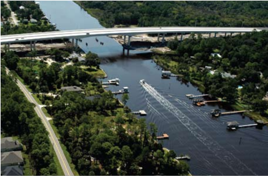
The Palm Valley Bridge over the St. John River in Florida uses spliced, post-tensioned concrete I-girders for the main span of 290 ft.
