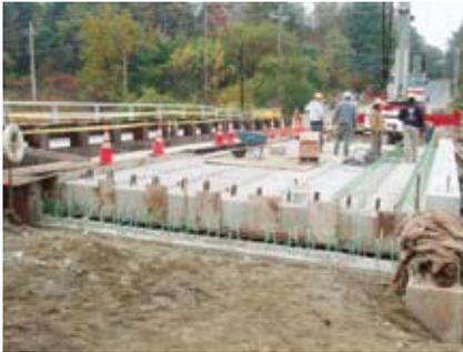
Railing anchor bolts were preset in the curb parapets prior to casting at the precasting plant.
