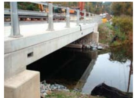
The adjacent slab beams were transversely post-tensioned at the abutments and midspan to help prevent longitudinal cracking along the shear keys.
