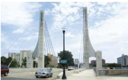
*Lane Avenue over the Olentangy River serves as a gateway to Ohio State University. The two-span, cable-stayed bridge limited environmental impacts, and the use of concrete allowed the contractor to complete the project 5 months early.*
