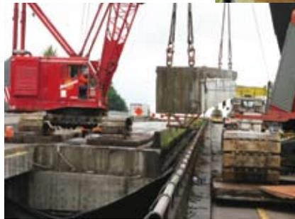
Good planning on the bridge program has allowed contractors to reuse precast concrete beams from detour structures. On a project near Eugene, 56 precast, prestressed box beams were salvaged from a detour structure and will be used on later projects.
