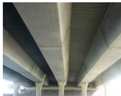
State Highway 52 over I-25: 322 ft long, 3 spans, 190-ft-long maximum span.
