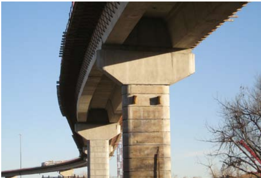
I-270 Ramp over I-76: 2282 ft long, 230-ft-long maximum span, 764-ft-minimum radius.
