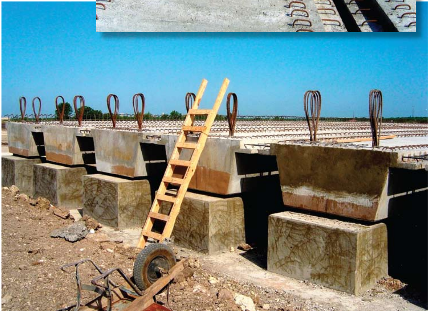
Beams were preassembled for casting the deck.
