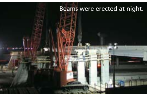
Pretopped U-beams were joined in the field with longitudinal and transverse closure placements.
