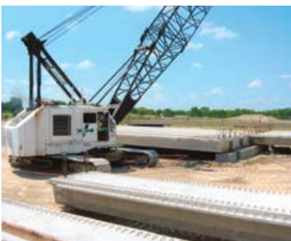
Beams were preassembled for casting the deck.
