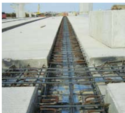
Pretopped U-beams were joined in the field with longitudinal and transverse closure placements.
