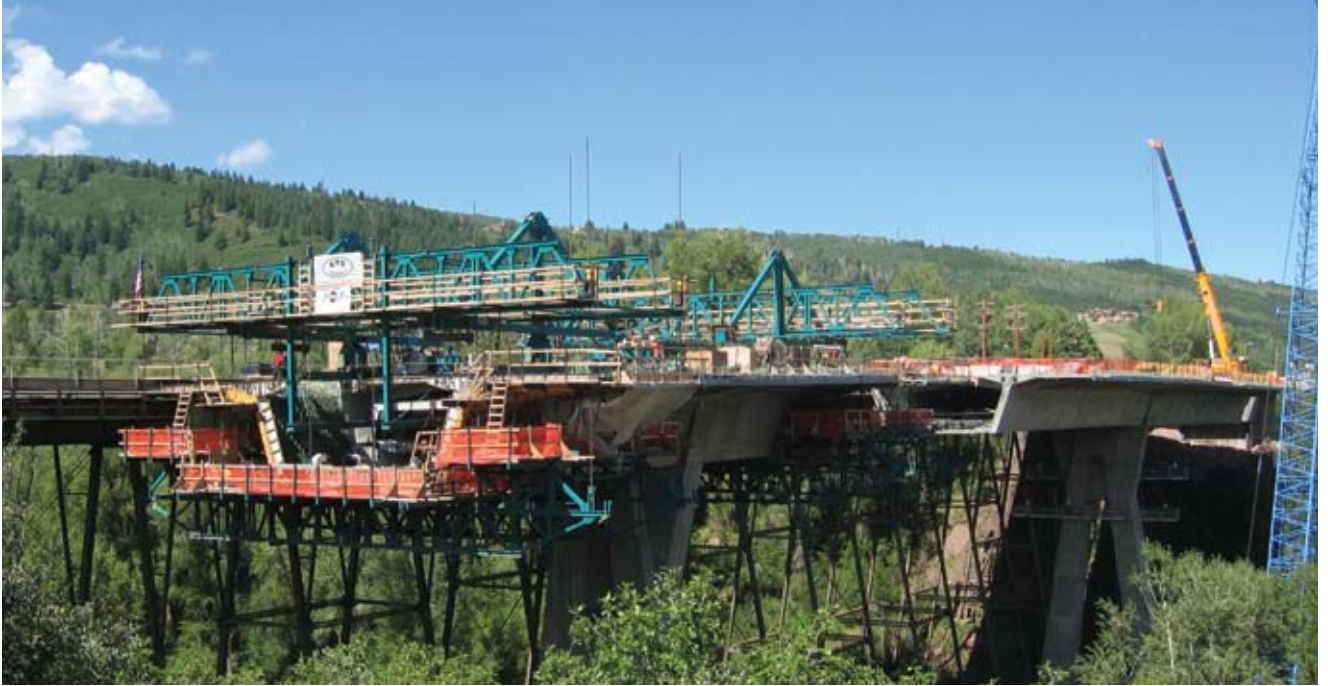
Overhead construction using form travelers continues on the second cantilever.
