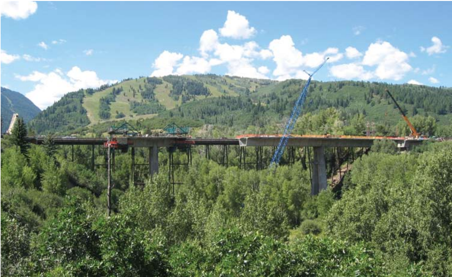
Overhead construction using form travelers continues on the second cantilever.
