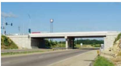
The Route 100 precast box beam bridge provides a shallow structure depth over I-44 near St. Louis, Mo. Photo: MoDOT.
