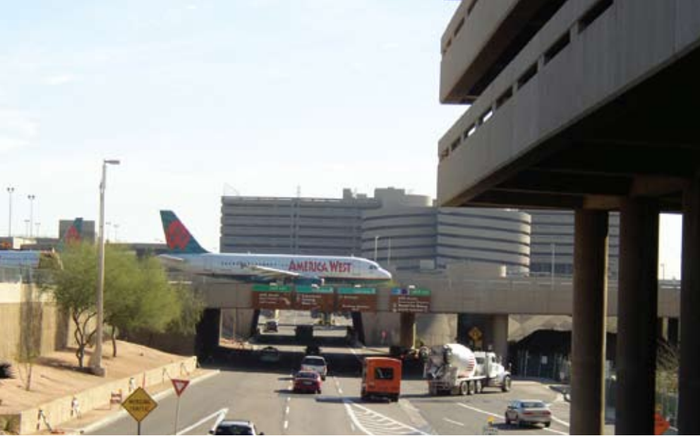
The structure was designed to support a gross aircraft weight of 1.5 million lb, plus a 30 percent impact factor. Photo: HDR Inc.
