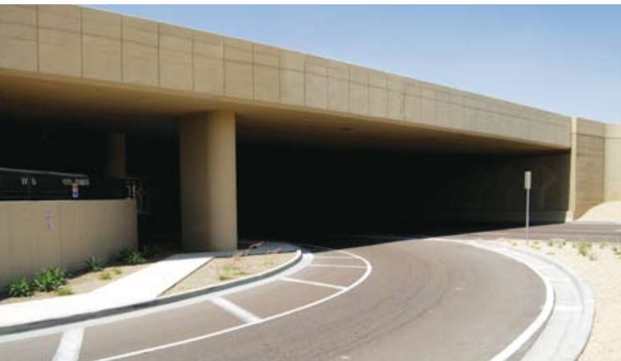
A five-span, cast-in-place, post-tensioned box girder bridge carried the taxiway across Sky Harbor Boulevard at the Sky Harbor International Airport. Photos: Richard Strange.
