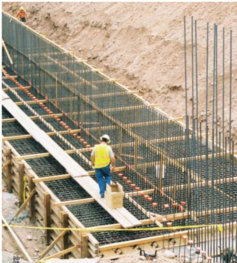
Inspector checking rebar placement for abutment 1.
