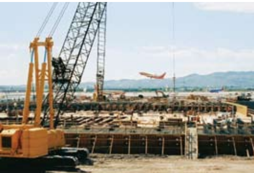
Deck concrete placement was carefully sequenced longitudinally and transversely. Photo: HDR Inc.
