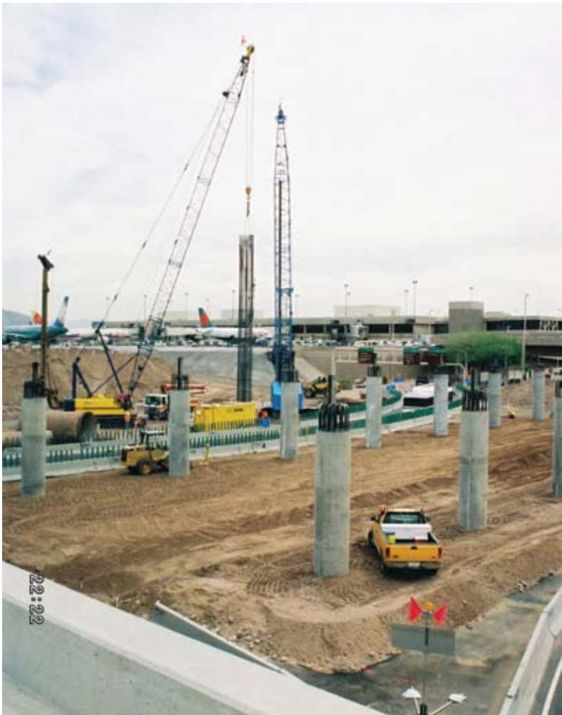
Eastern view of completed pier 2 and 3 columns. Photo: HDR Inc.
