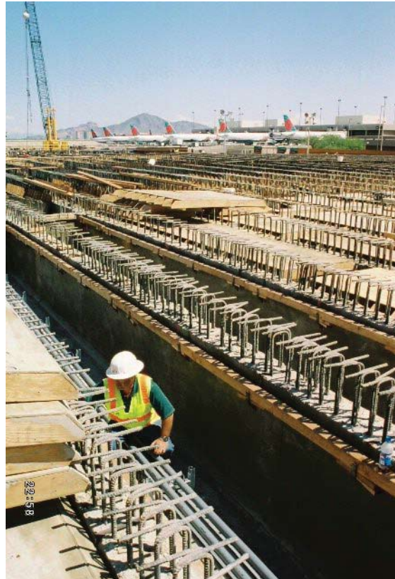
Worker with deck rebar.
