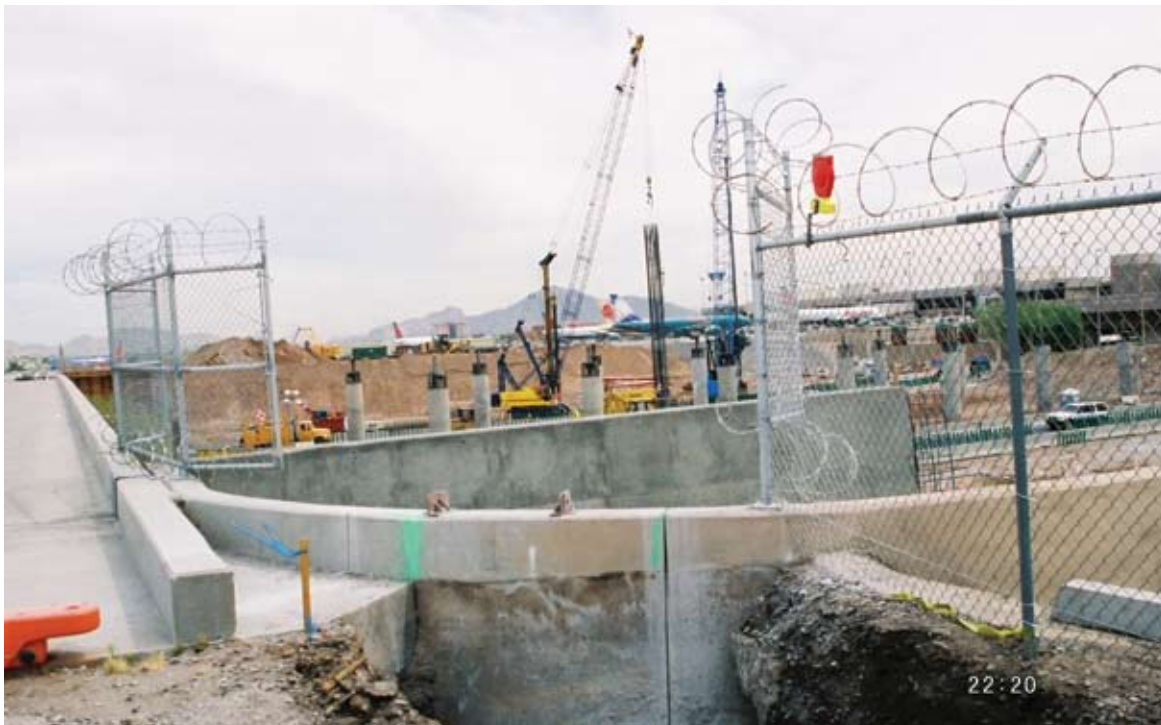
Northeast view of rebar cage set in caisson pier.
