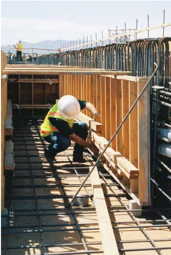
Worker with deck rebar.
