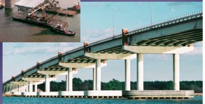
Mattaponi River Bridge - Virginia Lightweight concrete deck and long-span spliced girders.
