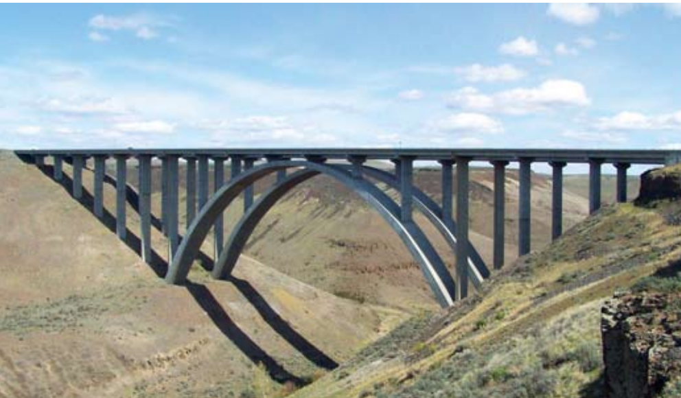
The Selah Creek Fred G. Redmond Bridges on I-82 near Yakima opened in 1971.
