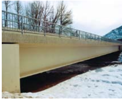
The Twisp River Bridge spliced "Super Girder."
