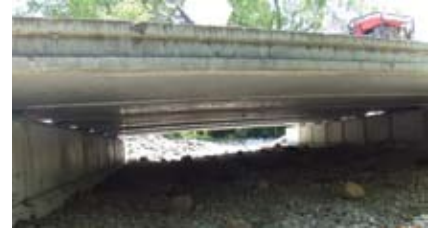
A culvert-replacement project over Lackamas Creek reused bridge slabs obtained from the City of Olympia, where they had been used for a temporary bridge.
