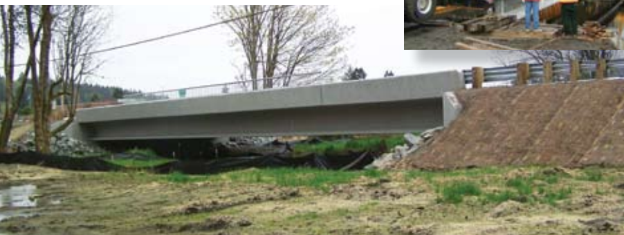
Old Highway Bridge No. O-9, originally built in 1923, was replaced in 2007 with a 110-ft-long, 42-ft-wide precast, prestressed concrete bridge.
