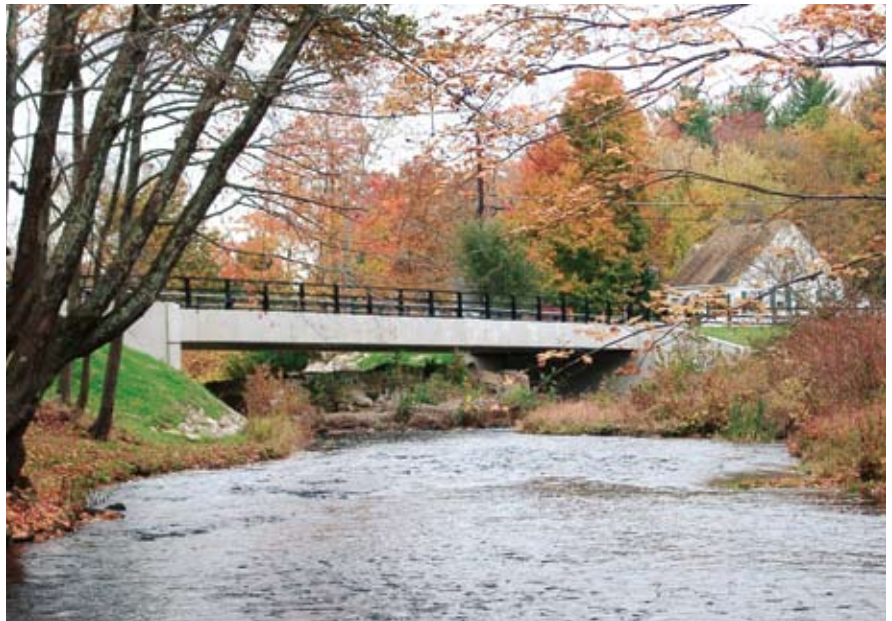
The Mill Street Bridge in Epping, New Hampshire, was built in only 8 days to minimize construction-related traffic delays and improve work zone safety.
