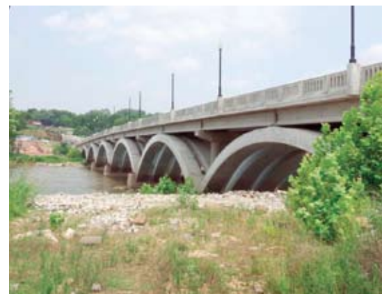
Four pairs of precast post-tensioned arch ribs of the Dan River Bridge replicate the existing Luten spandrel arch.
