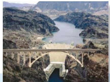
The Hoover Dam Bypass Bridge features a composite concrete deck arch that complements the nearby dam and spans the 800-ft-deep Colorado River gorge. The 1914-ft-long bridge will be the longest concrete arch span in the United States when completed. Photos: T.Y. Lin International.
