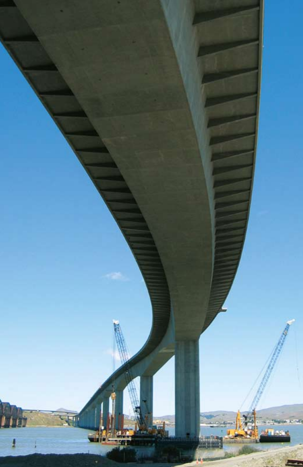
The new Benicia-Martinez Bridge is built of sand-lightweight concrete, cast-in-place segments with span lengths of 418 to 659 ft. Photo: T.Y. Lin International.
