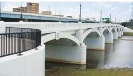
The Washington Street Bridge over the Great Miami River is a three-lane, seven-span, precast, prestressed concrete box beam bridge with precast concrete arch segments and cast-in-place concrete wall piers. It has 10-ft-wide sidewalks with decorative lighting above and below the bridge.
