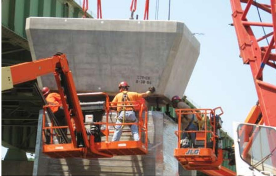
Ironworkers align the couplers for the post tensioning bars as they set the precast concrete column cap segment at pier 7. Photo: Renata Magoc.
