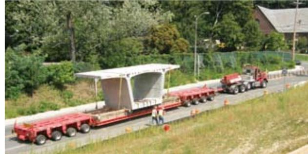
To protect the waterway near the site, precast concrete segments were barged from the precaster's plant in Cape Charles, Va., to a location several miles from the project and then hauled by specialized trailers to the site.
