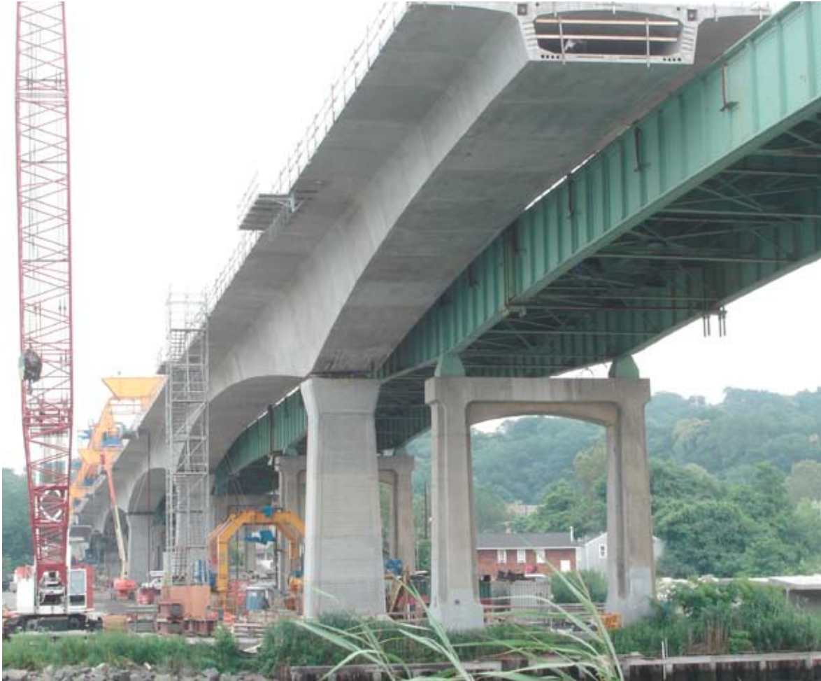
Tapered pier columns create a new visual appeal for the Roslyn Viaduct. The near end will tie into the east abutment. Photo: Rich Lorenzen.
