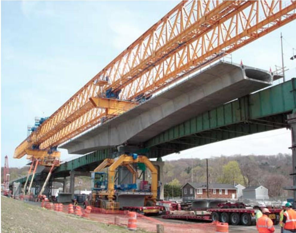
A completed cantilever section over pier 5. In the foreground, a straddlecarrier moves segments into position on the ground. Photo: Rich Lorenzen.
