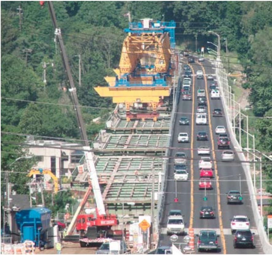
After the north side of the bridge was constructed, the gantry crane was shifted to the south to remove the steel frame of the existing bridge. Photo: Rich Lorenzen.
