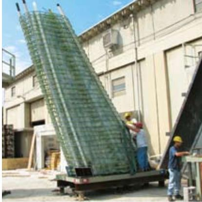
(Right Photo) Inclined, voided, precast concrete column being handled in the casting yard.
