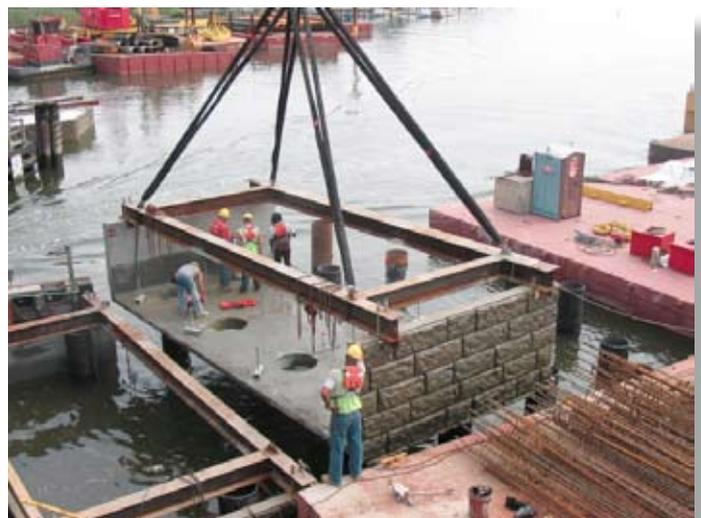
Precast cofferdam section being lowered into place.
