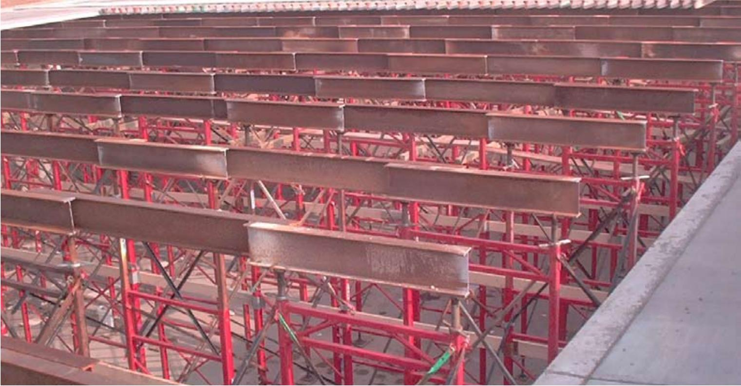
Falsework for the cast-in-place slab was put in place after completing the end bents and MSE walls.
