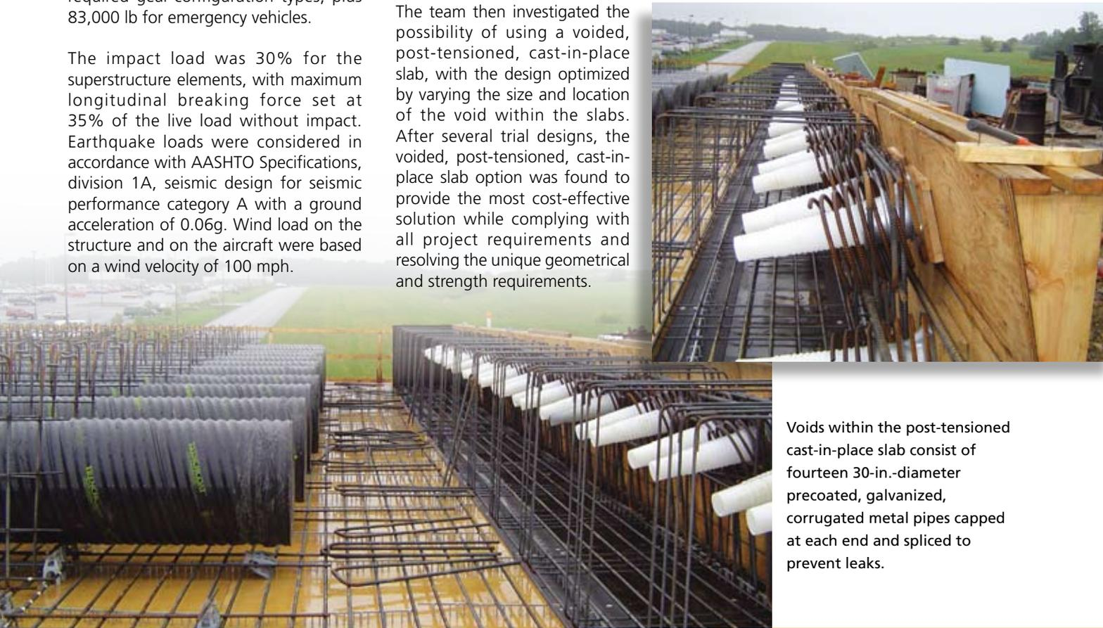
Voids within the post-tensioned cast-in-place slab consist of fourteen 30-in.-diameter precoated, galvanized, corrugated metal pipes capped at each end and spliced to prevent leaks.
