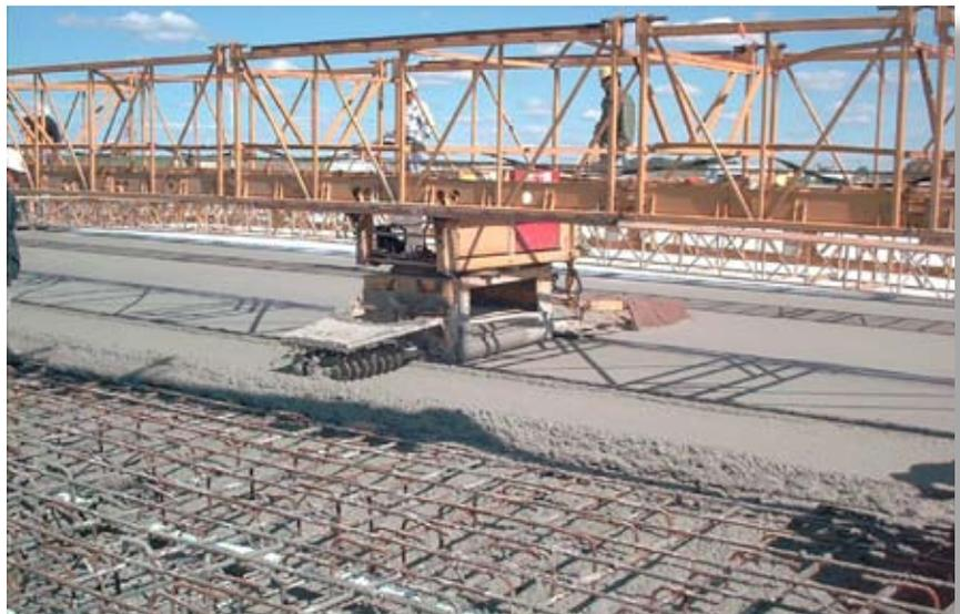
The final lift of concrete for the voided slab is consolidated and screeded.
