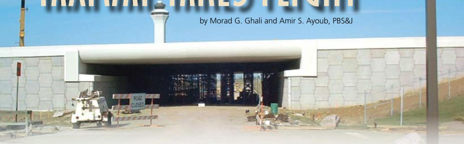
The new taxiway at the Cincinnati/Northern Kentucky International Airport features a single post-tensioned, cast-in-place span to support the required loading and maximize clearance above the roadway. Photos: PBS&J.
