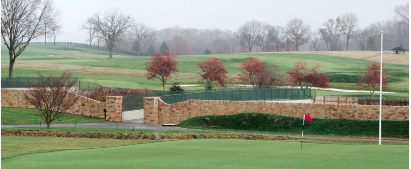
Piers from the bridge are textured and stained to complement the landscape from the golf course at Oakmont Country Club. Photo: © FIGG.
