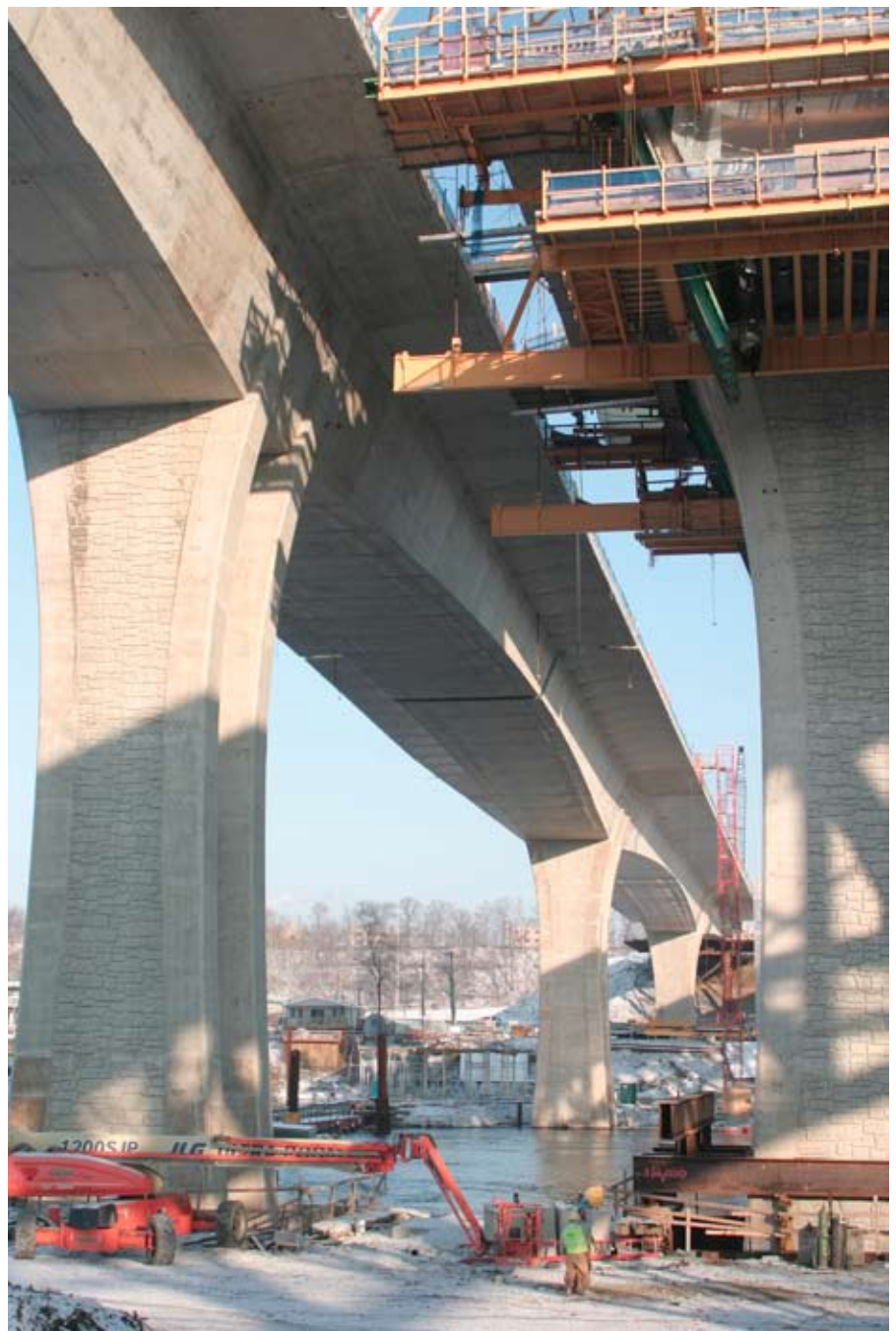
The variable depth superstructure creates an arching form over the Allegheny River. Photo: © FIGG.
