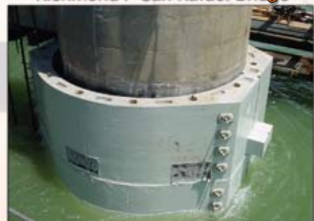
Richmond / San Rafael Bridge
