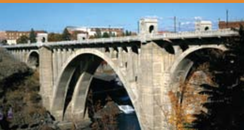
Monroe Street Bridge Rehabilitation Spokane, Washington 2006 Gold Award, Engineering Excellence, ACEC Washington
