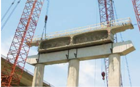
End segments for the main spans were precast on the footing below their final location and lifted into position. Photo: Traylor Bros.
