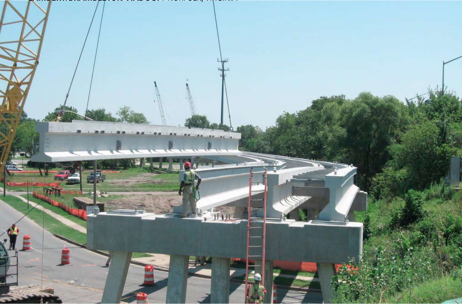
Girder erection in open deck spans. Photo courtesy of HRT.
