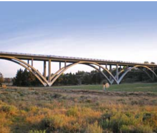
Maple Avenue Bridge, Redmond, Ore.
