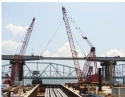
The $50-million Rigolets Pass Bridge replaced a steel-truss swing-span structure with a high-level spliced girder concrete bridge that provided 65 ft of vertical and 200 ft of horizontal clearance for marine traffic.
