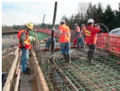
A cast-in-place deck was used for the walkway (Deck pour span six).
