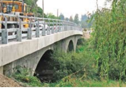
South Slough Bridge 91. This bridge has won several local and national awards for innovative design and construction techniques including the use of lightweight cellular concrete. It was a winner in the 2008 Portland Cement Association Bridge Awards program. For more information visit www1.co.snohomish.wa.us and search "Bridge 91."
