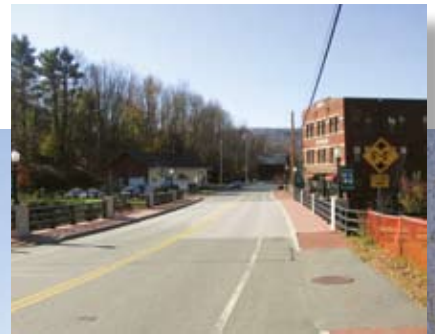
Completed Main Street Bridge with historic mill in the background.
