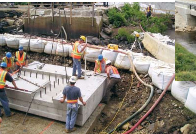
Placement of the first precast footing segment in NHDOT's first entirely precast bridge in Epping.
