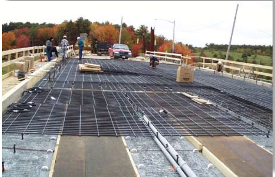
Workers begin installation of CFRP grids in Rollinsford.
