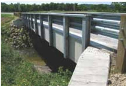
An adjacent precast, prestressed concrete box beam bridge with side-mounted metal traffic rails in Monroe County, Wis.
