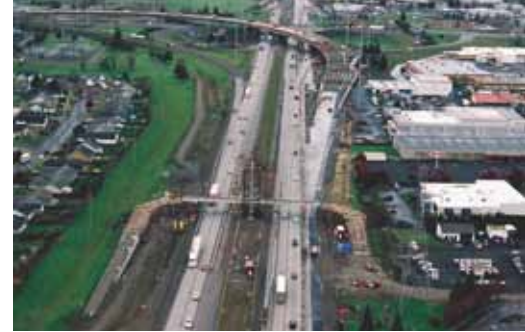
Location of the pedestrian bridge in context of the Beltline Interchange Improvement Project. Photo: Oregon Department of Transportation.
