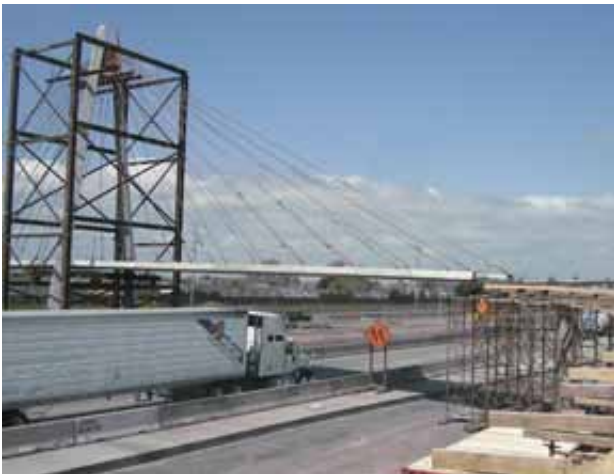
Daytime traffic under balanced cantilever main spans. Photo: OBEC Consulting Engineers.
