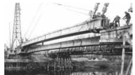
Erection of the partially assembled segments of the Luzancy Bridge in 1946.
