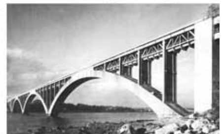
Plougastel Bridge with 610-ft span.
