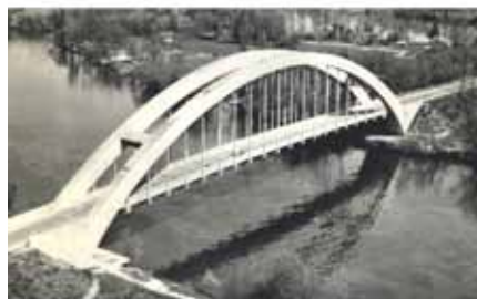
Saint-Pierre-du-Vauvray Bridge with 430-ft span.
