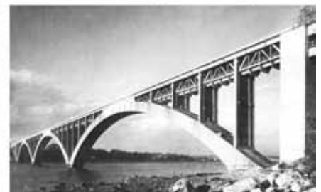
Plougastel Bridge with 610-ft span.
