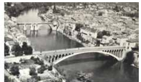
Villeneuve-sur-Lot Bridge with 315-ft span.
