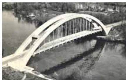
Saint-Pierre-du-Vauvray Bridge with 430-ft span.
