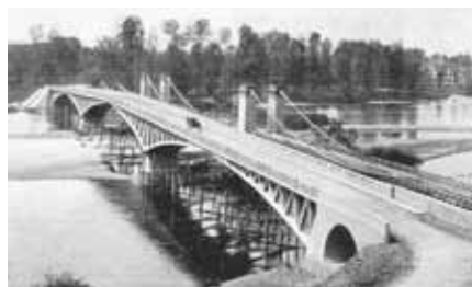
Veudre Bridge with 238-ft span.
