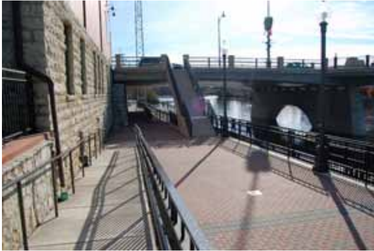
New stairs for bridge and river walk access on northeast corner of Wilson Street. Photo: H.W. Lochner Inc.
