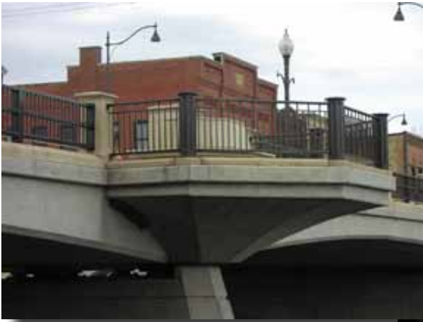
The river outlook showing how the facets of the soffit frame into the facets of the pier. Photo: Henry G. Russell Inc.
