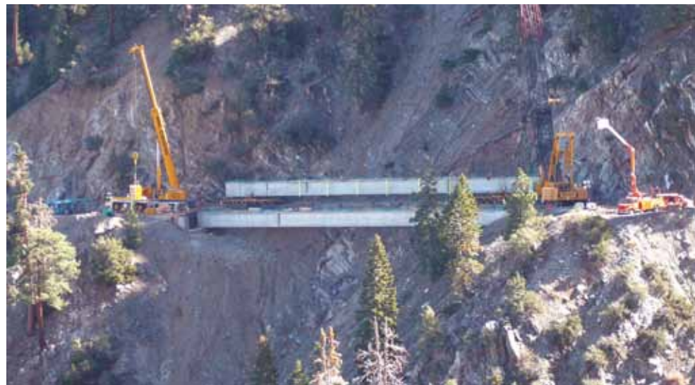
The temporary haul road crosses the uphill end of the abutments to allow delivery of materials including the assembled girders. Note the braced forms and bridge over the forms. Once girders were delivered, the road was removed and the full abutment unearthed.
