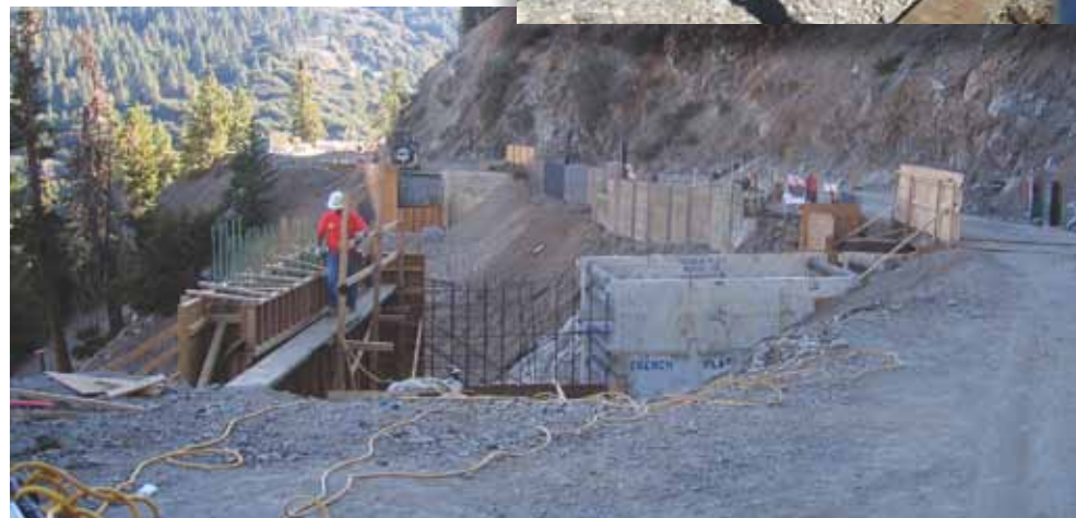
The temporary haul road crosses the uphill end of the abutments to allow delivery of materials including the assembled girders. Note the braced forms and bridge over the forms. Once girders were delivered, the road was removed and the full abutment unearthed.
