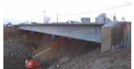
The Wheeler Road Bridge No. 244 was a five span structure replaced in February 2010 with a 165-ft-long single-span deck bulb-tee girder. Photo: Larry Maine, Grant County.
