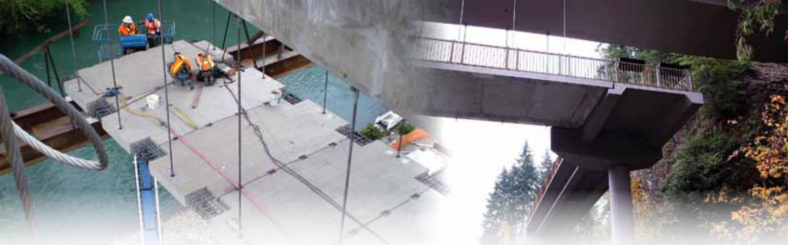
The pedestrian bridge features 56 precast concrete deck segments below the main bridge and four deck bulb-tee approach girders along the river bank to transition to the Olympic Discovery Trail.
