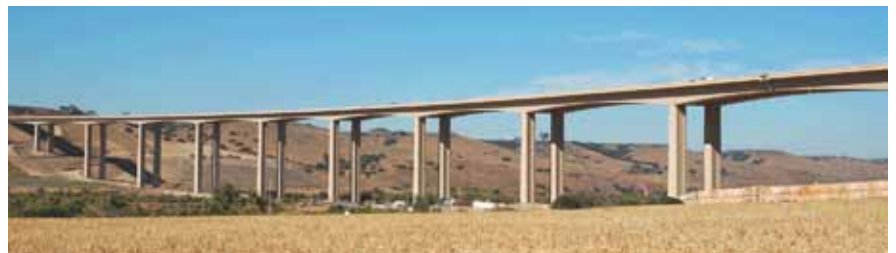
The 3325-ft-long Otay River Bridge in San Diego, Calif., features twin variable-depth box girders connected by a transverse diaphragm at the piers and cast-in-place slab along the bridge's centerline. The 640 trapezoidal box girder segments, erected via the balanced-cantilever method, used a self-launching overhead gantry to minimize site disruptions.
