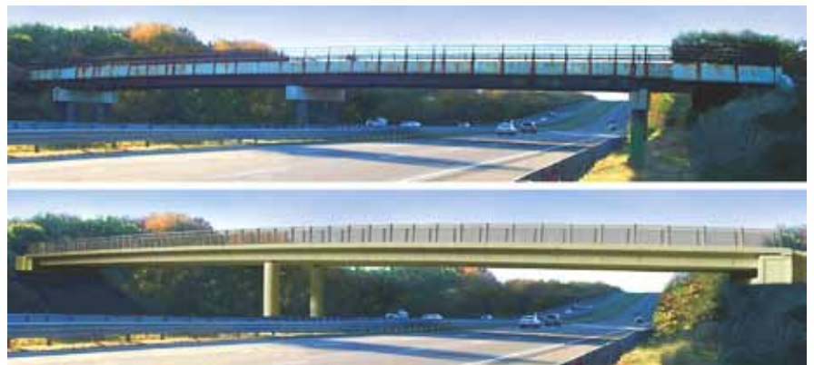
The DCR Access Road over Route 24 Bridge in Randolph, Mass., now underway, uses two large edge girders as roadway barriers, reducing materials and increasing vertical clearance. The low profile adds 2.5 ft to the vertical clearance without altering the approach grade.
