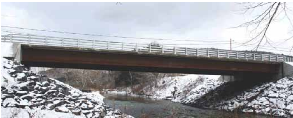
State Route 23 over Otego Creek near Oneonta, N.Y., features conventional precast concrete deck panels with extended reinforcement spliced in 6-in.-wide connections using UHPC. Photo: FHWA.
