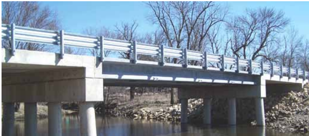
Jakway Park Bridge near Aurora, Iowa, is the first project to use the optimized pi girder. It is 33 in. deep and spans 87 ft. Photo: FHWA.
